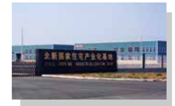
华东产业示范园(连云港) 江苏省装配式建筑部品构件生产基地 East China Industry Demonstration Park (Lianyungang) Prefabricated Building Component Production Base in Jiangsu province
